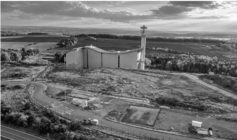
Figure 4. Waste incineration plant in Chotíkov
