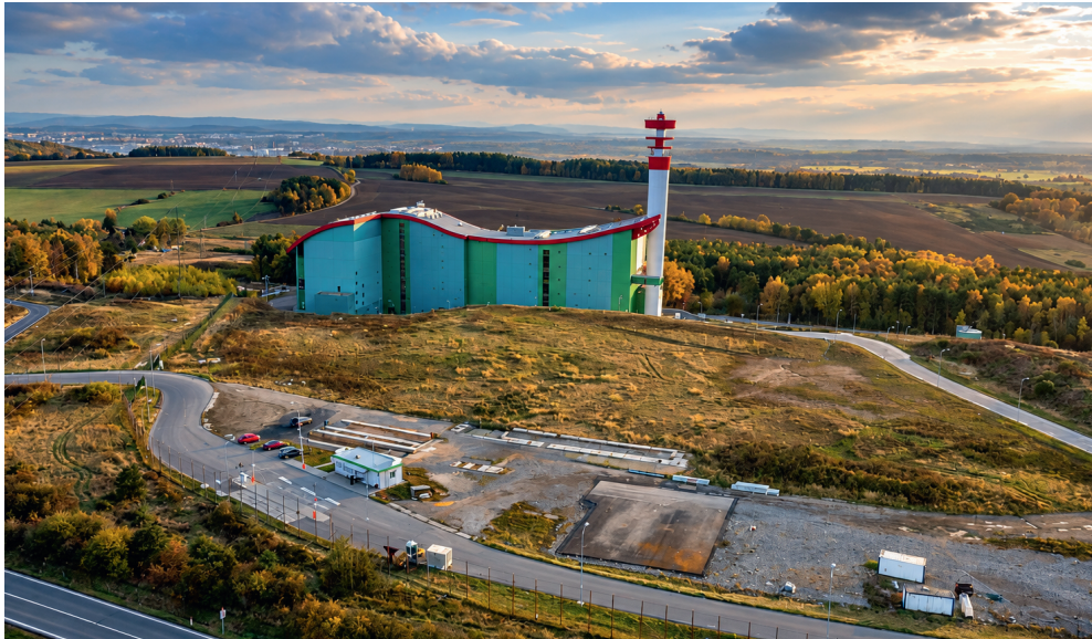
Figure 4. Waste incineration plant in Chotíkov
