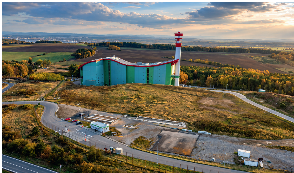
Figure 4. Waste incineration plant in Chotíkov
