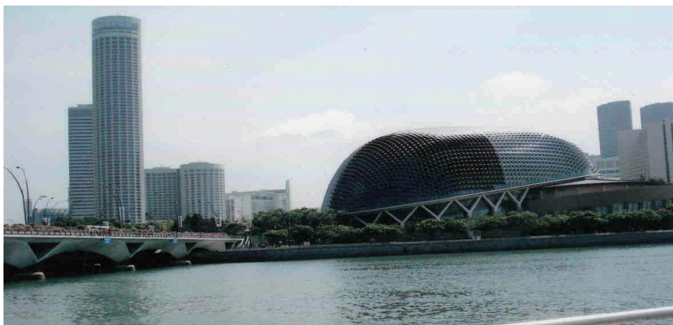
Fig. 3. New Singapore theatre – one of the latest buildings. It has an original mirror roof (the author’s photo)
